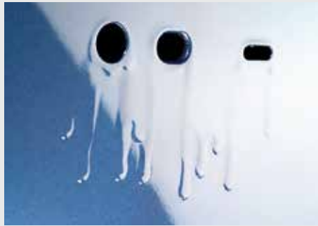
Removing paint runs
